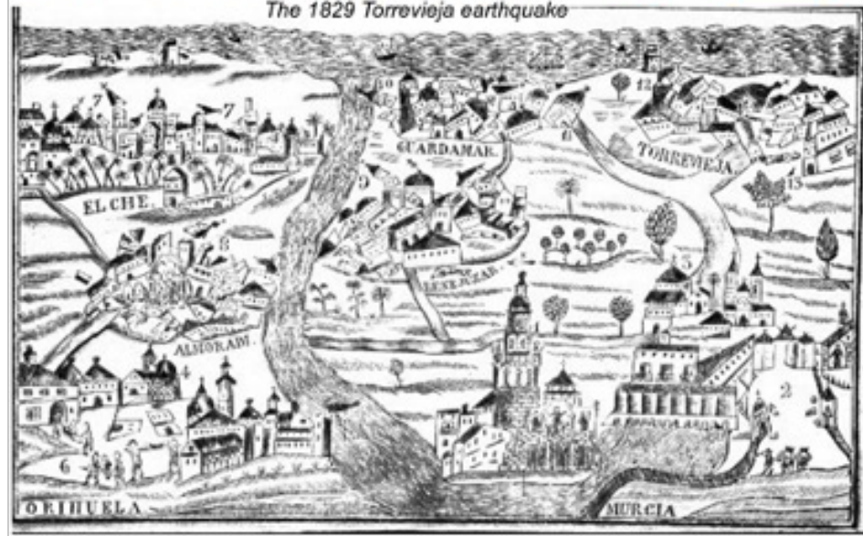
The 1829 Torrevieja earthquake
